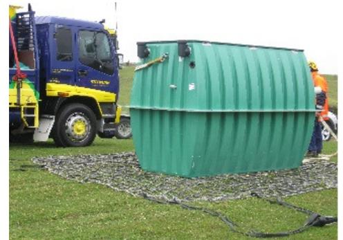
The AX15 has lifting eyes for ease of loading/unloading; the Skyworks team opted to use the net for extra safety
