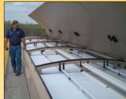
▲ The AX-Mobile uses textile sheets in a packed bed media filter. It can treat blackwater and grey-water to a level where effluent can be reused for surface or subsurface irrigation or dust control (as regulations permit).
