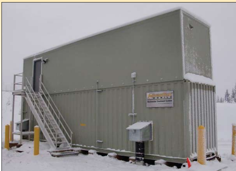
▲ The remote telemetry control panel for an AX-Mobile Treatment System is typically installed at the end of the unit and pre-wired.
