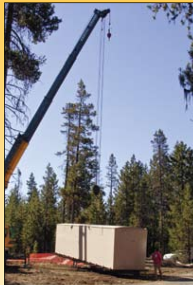
▲ The largest AX-Mobile™ unit weighs 10,000 lbs (4,536 kg), and can be transported by truck, rail, cargo container, or helicopter.
