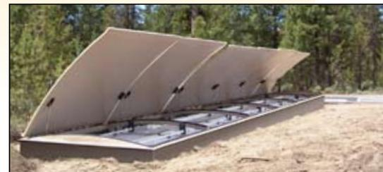
This full-sized AX-Max wastewater treatment system was recently installed at a 50-site campground in the LaPine, Oregon State Park.
